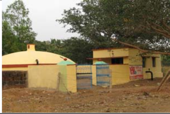
BHUSANDAPUR PUMP HOUSE
